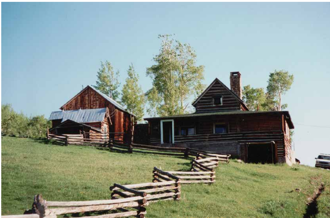
Bunkhouse and house in Routt County
